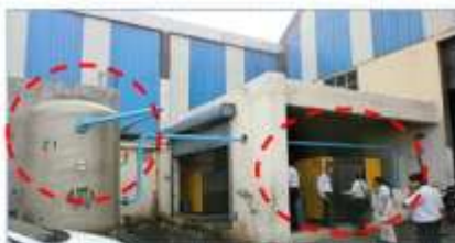
e.g.1: Installation of new receiver and new air compressors (not inverter type)
